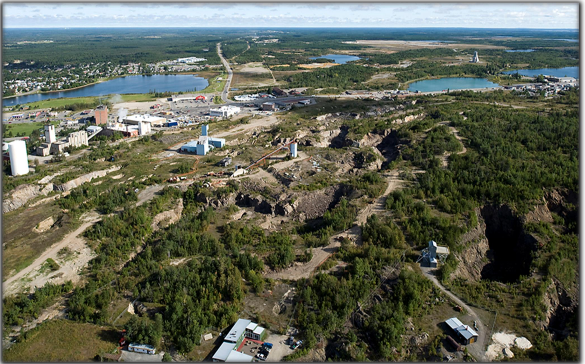
Aerial Image of Hazards
