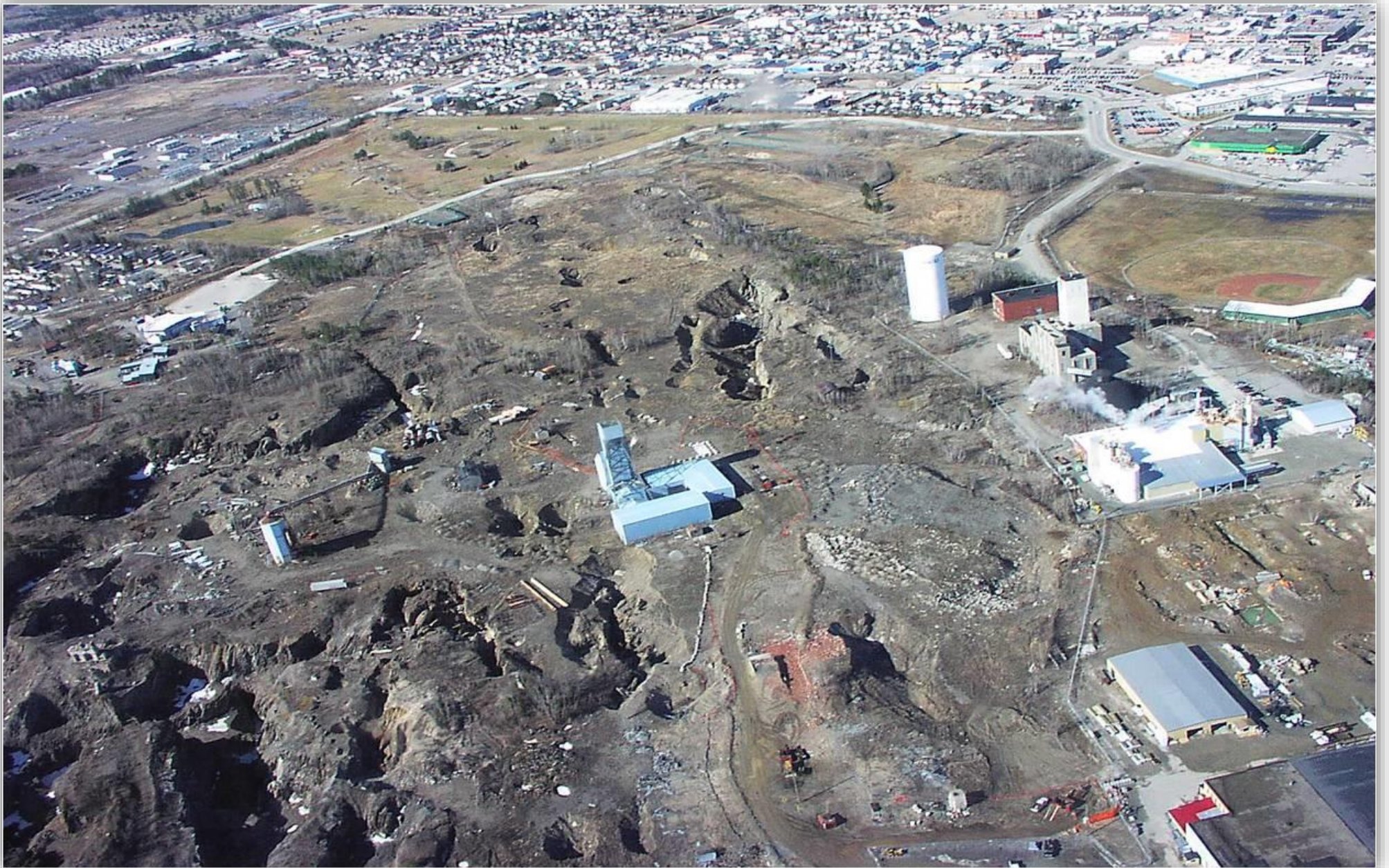
Aerial Image of Hazards
