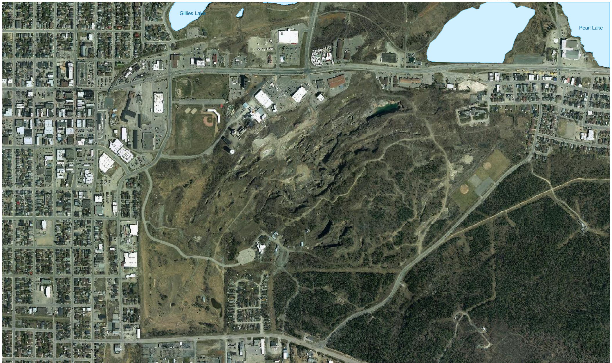
Aerial View of Hazards
