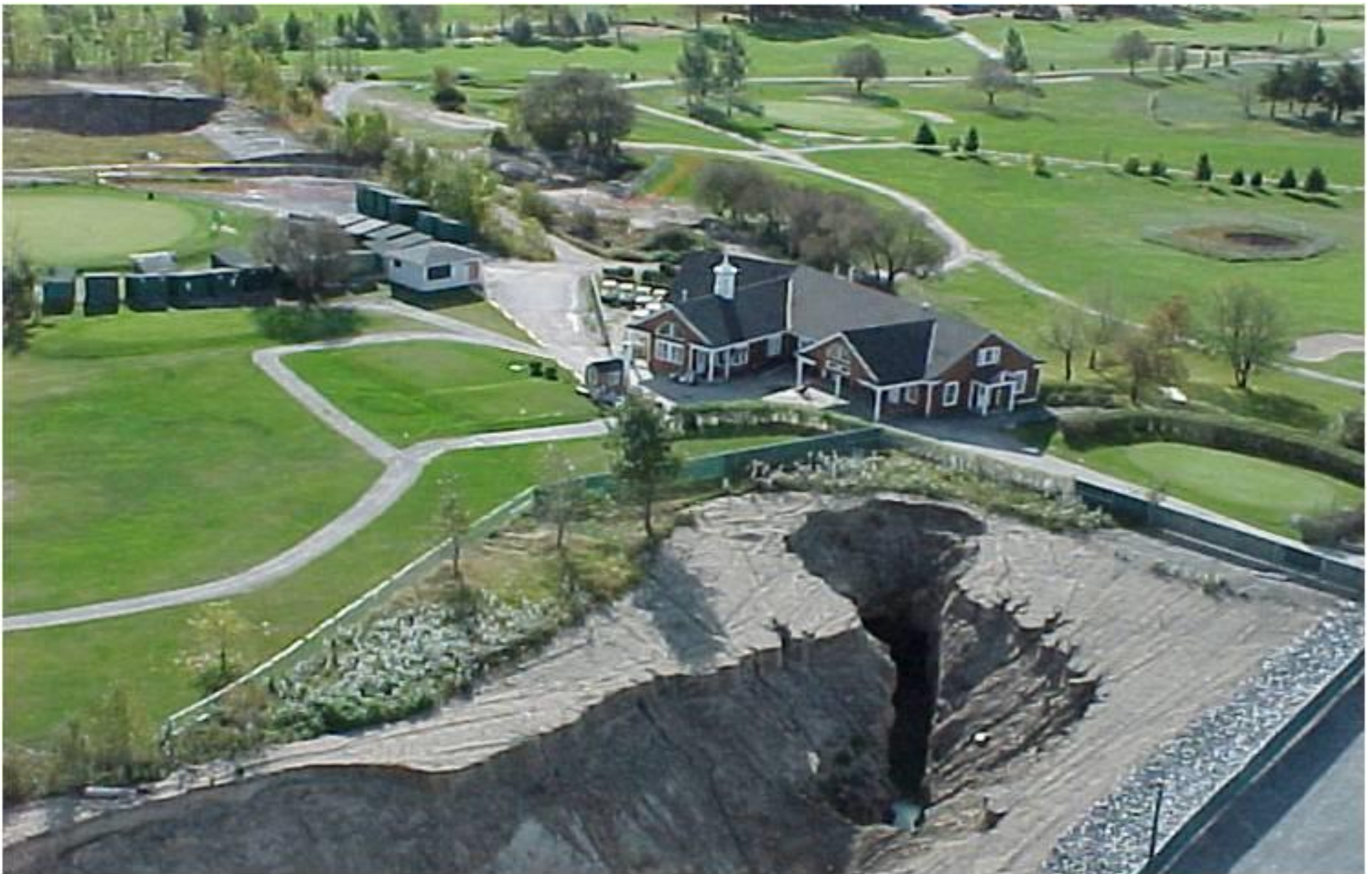
Subsidence - Golf Course
